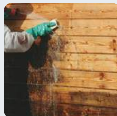
Let it work for 5 minutes, then rinse thoroughly with water
