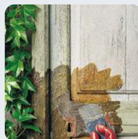
On paint, let it work for at least 30 minutes per coat.
