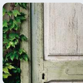
Apply DILUNETT® on to dry wood.
