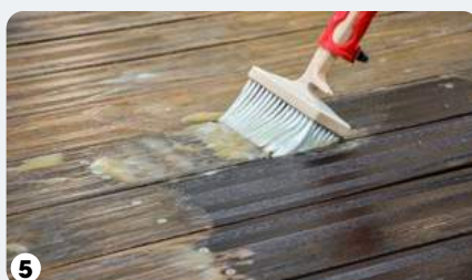
Apply NET-TROL®* onto wet wood to neutralise.
